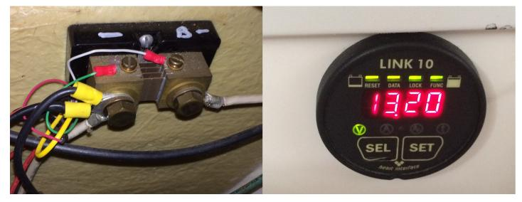
Above is the shunt resistor as installed. The small white and green wires are the sense wires that connect to the battery monitor. The heavy white wire goes to the battery negative and the others are all negatives from various equipment.
